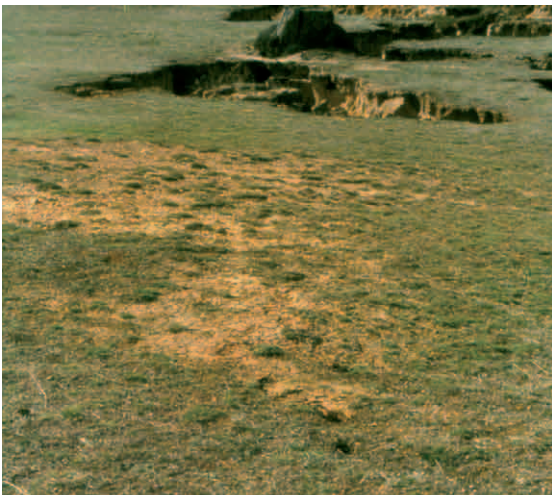
Figure 10 Dispersible soil emerging from tunnel erosion
