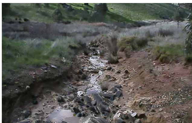
Figure 13: A correctly constructed spillway. Photo: A. Cole.
