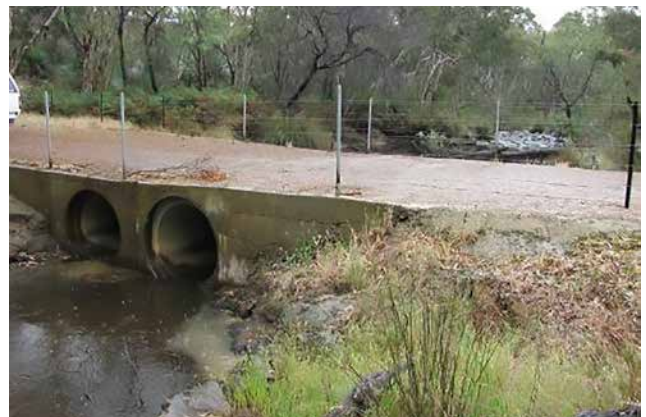
Figure 5: Correctly designed and installed culvert creek crossing Photo: A. Cole
