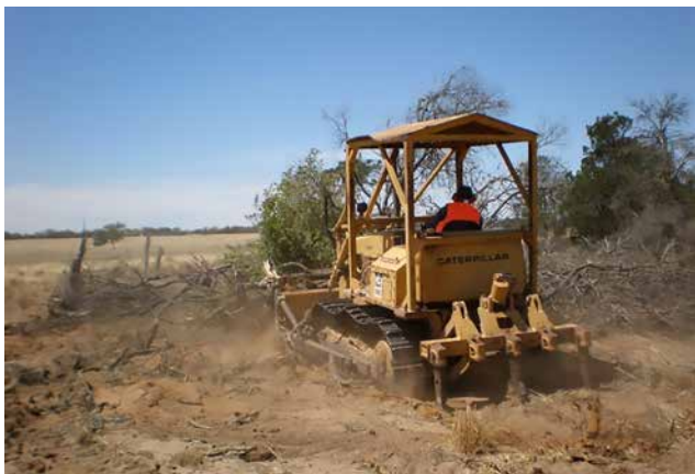
Figure 3: Tractor with 3 tines ripping a rabbit warren Photo: S. Edwards
