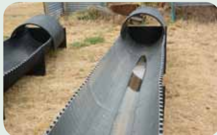
Top image: Watering point riser. Middle: Solar panel and pump to service piping. Bottom: Portable watering trough. Photos: G. Johnson
