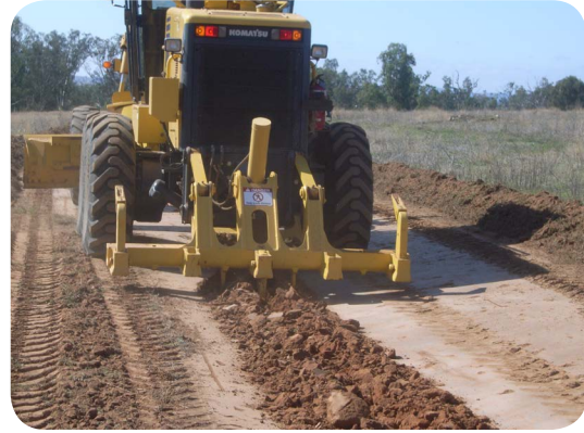
Cultivation at half depth in the first pass.
