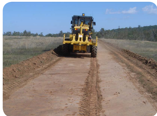
Scalping using a grader removes approximately 75 mm of soil including much of the soil seed bank, which is windrowed to the side. In this example, a gentle spoon drain or furrow is created that harvests rainfall from the surrounding area to the centre providing long lasting weed control and water harvesting in one action. This high disturbance preparation method should be used very cautiously. Avoid sites prone to soil erosion such as duplex soils with a shallow sub-soil (B horizon) or sites with good native plant cover. It is best used in flat to gently sloping weedy sites with limited native groundcover.
