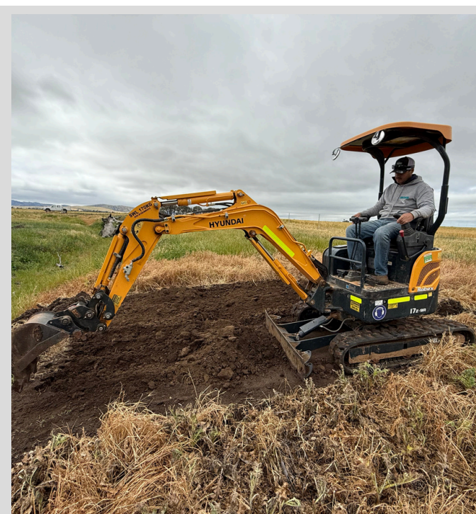
Mini excavator to scalping topsoil patches across the 16Ha site
